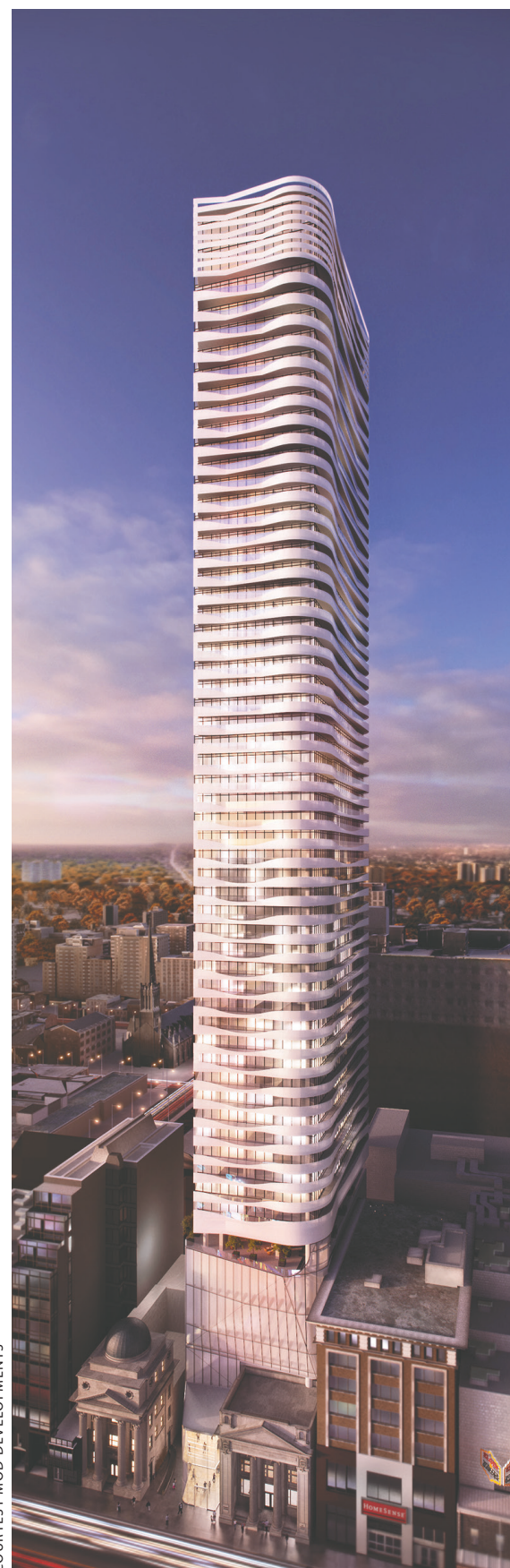
Massey Tower won the Building Industry and Land Development Association's high-rise project of the year award in 2013.
